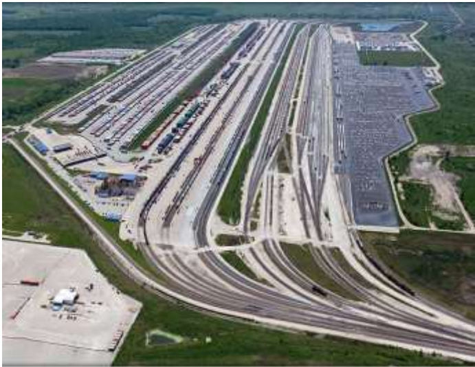
Figure 5 - BNSF Intermodal Terminal, Chicago, Illinois
