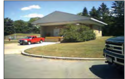
Pulaski's wastewater treatment facility. villagepulaski.org/
