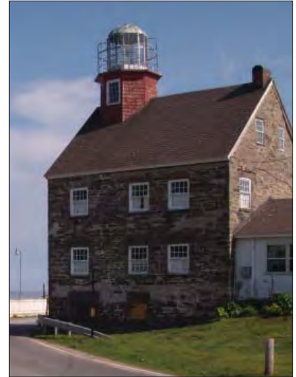
Selkirk Lighthouse, Summer 2008.
