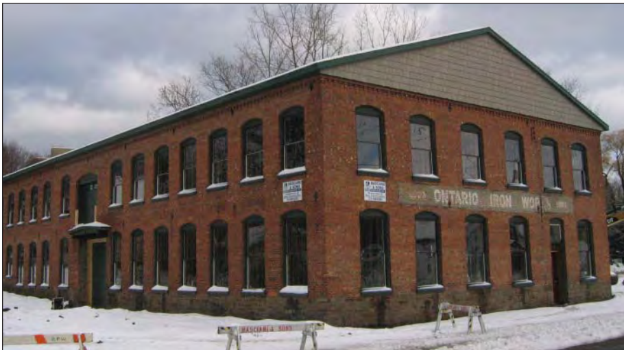
The Ontario Iron Works Foundry Building on Maple Avenue in the Village of Pulaski.
