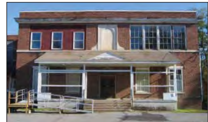
The former Pulaski School Annex (1926) building, in need of rehabilitation just beyond the Historic District in Pulaski.
