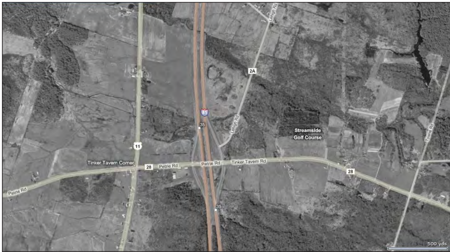
Satellite view of the Route 81 Tinker Tavern Interchange in Richland, NY. (source: Microsoft Corporation, NAVTEQ, Pictometry International Corporation, 2008).
