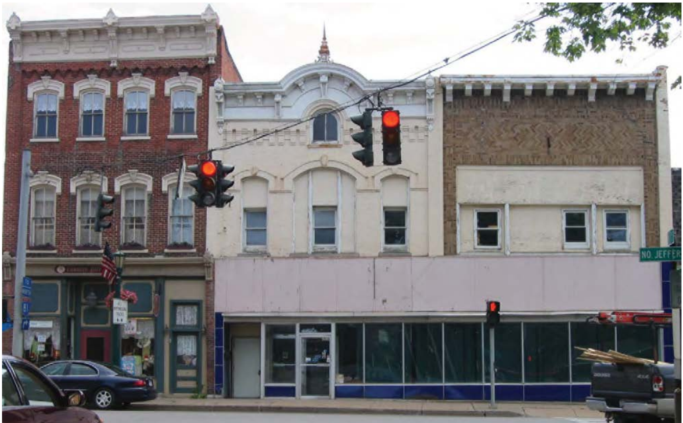
Existing conditions of the historic Jefferson Street buildings in 2008.
