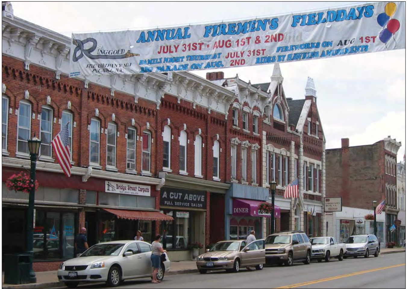
A row of nineteenth century buildings along Jefferson Street in the Historic District of the Village of Pulaski, NY
