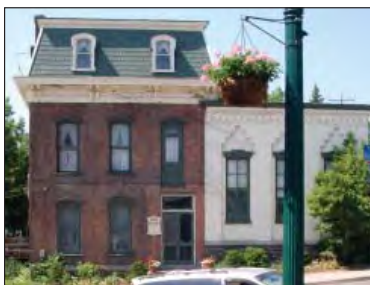
Salina Street in the Historic District, Pulaski, NY, 2008.
