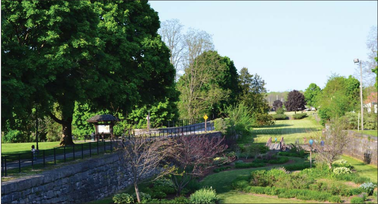
Former location of Erie Canal, Jordan
