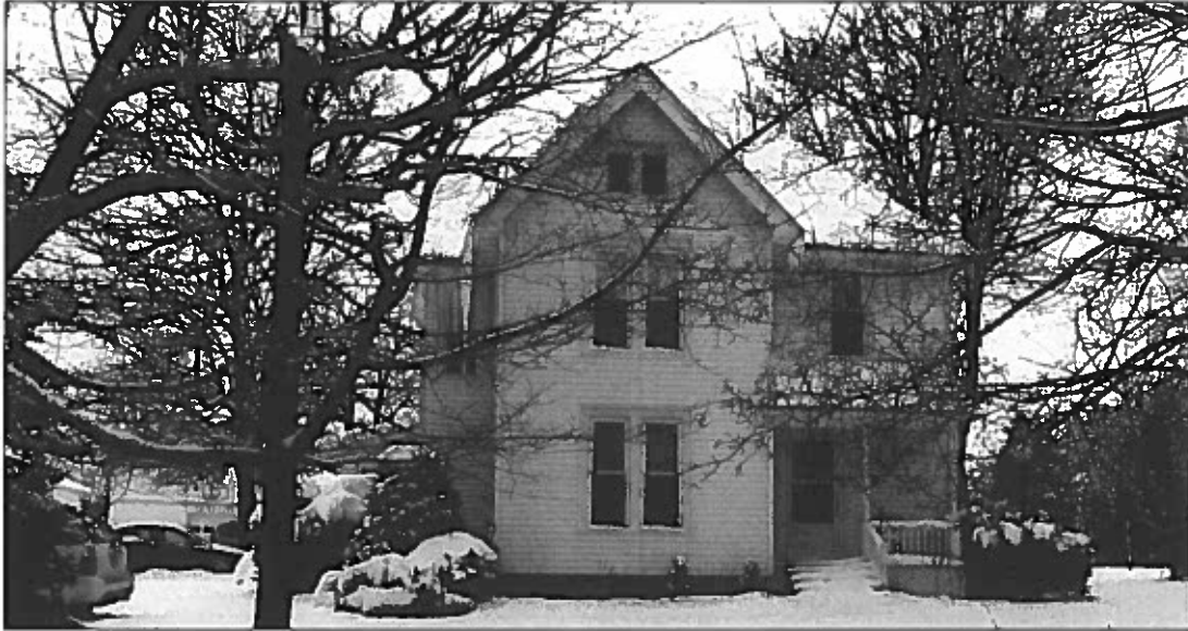
Front (north) elevation of parsonage with barn in far left background
