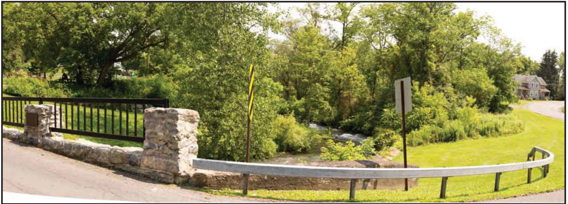
Site 14: West end of Crowhill Bridge, looking south
