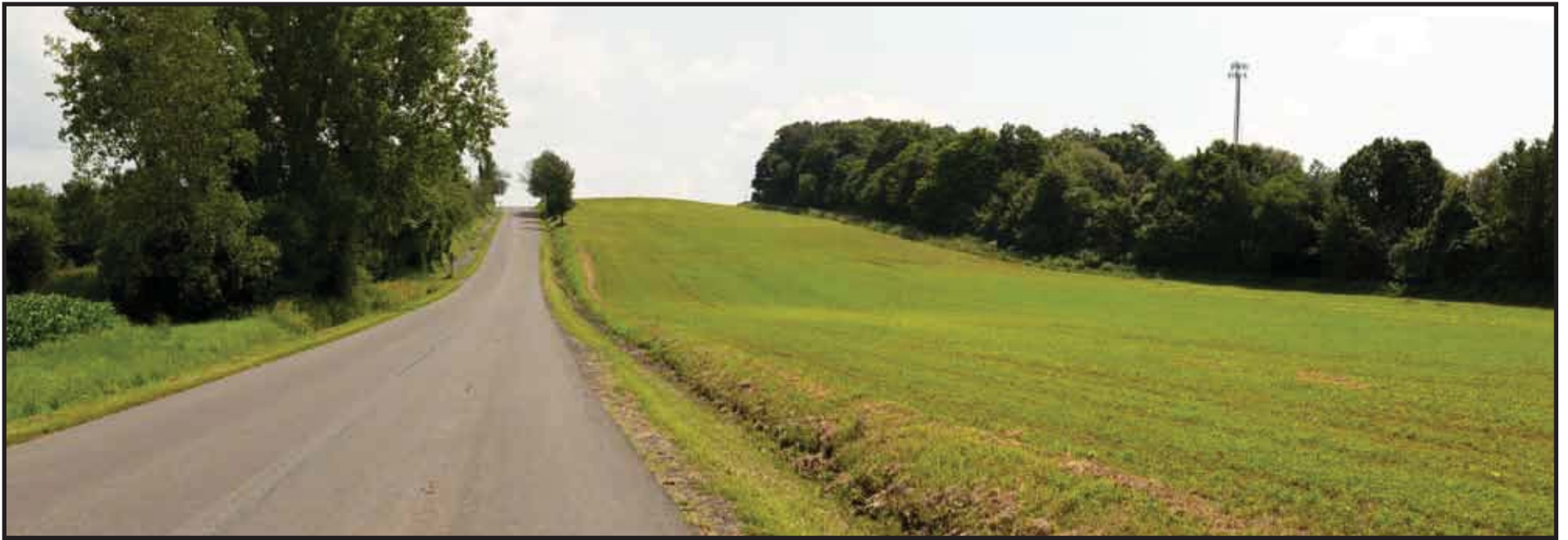
Site 11: 500 feet north of County Line Road / Sheldon Road intersection, looking south
